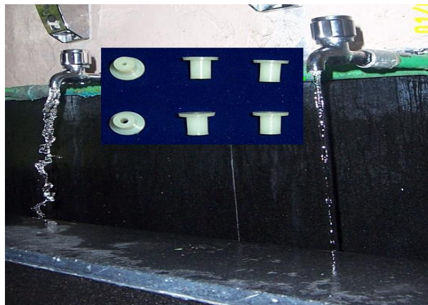
Water Taps 'With' and 'Without' Nylon Orifice Shown at the Centre are the Orifices Used
